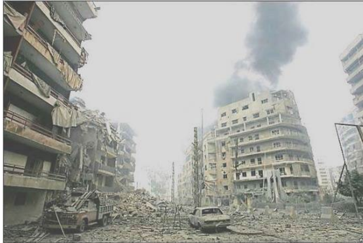
Figure 20: Example of MDZ-Like Blast Damage
